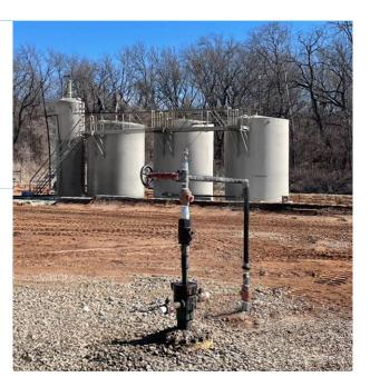
Permanent production facilities have been installed, comprising oil storage tanks, separator and flowlines and light crude oil with an API of 32 degrees is being sold. To date, over 3,000 barrels of oil have been produced and sold whilst testing.
